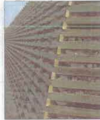
PLANTED TIMBER PERMACRIB WALL, WITH 1200MM HIGH TIMBER FENCE ABOVE
