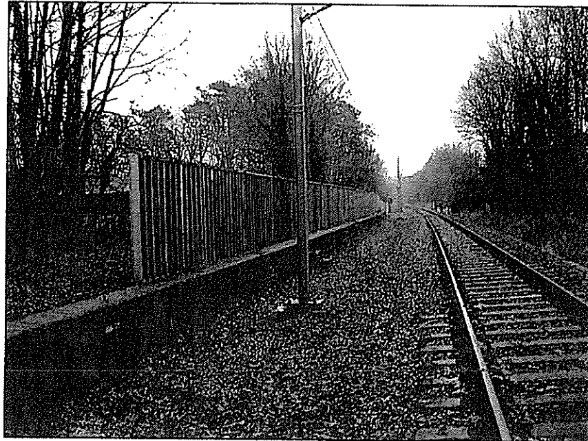
Figure 3.15: Noise Barrier from the Track Side
