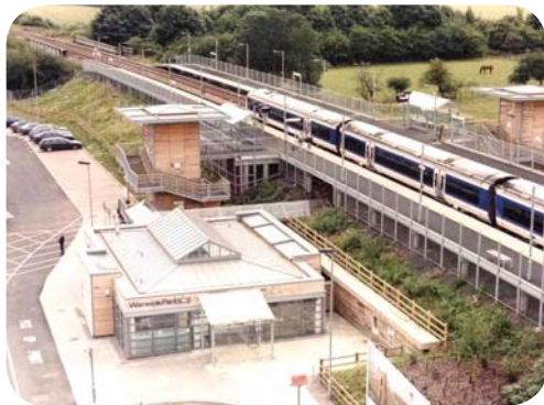
Warwick Parkway station
